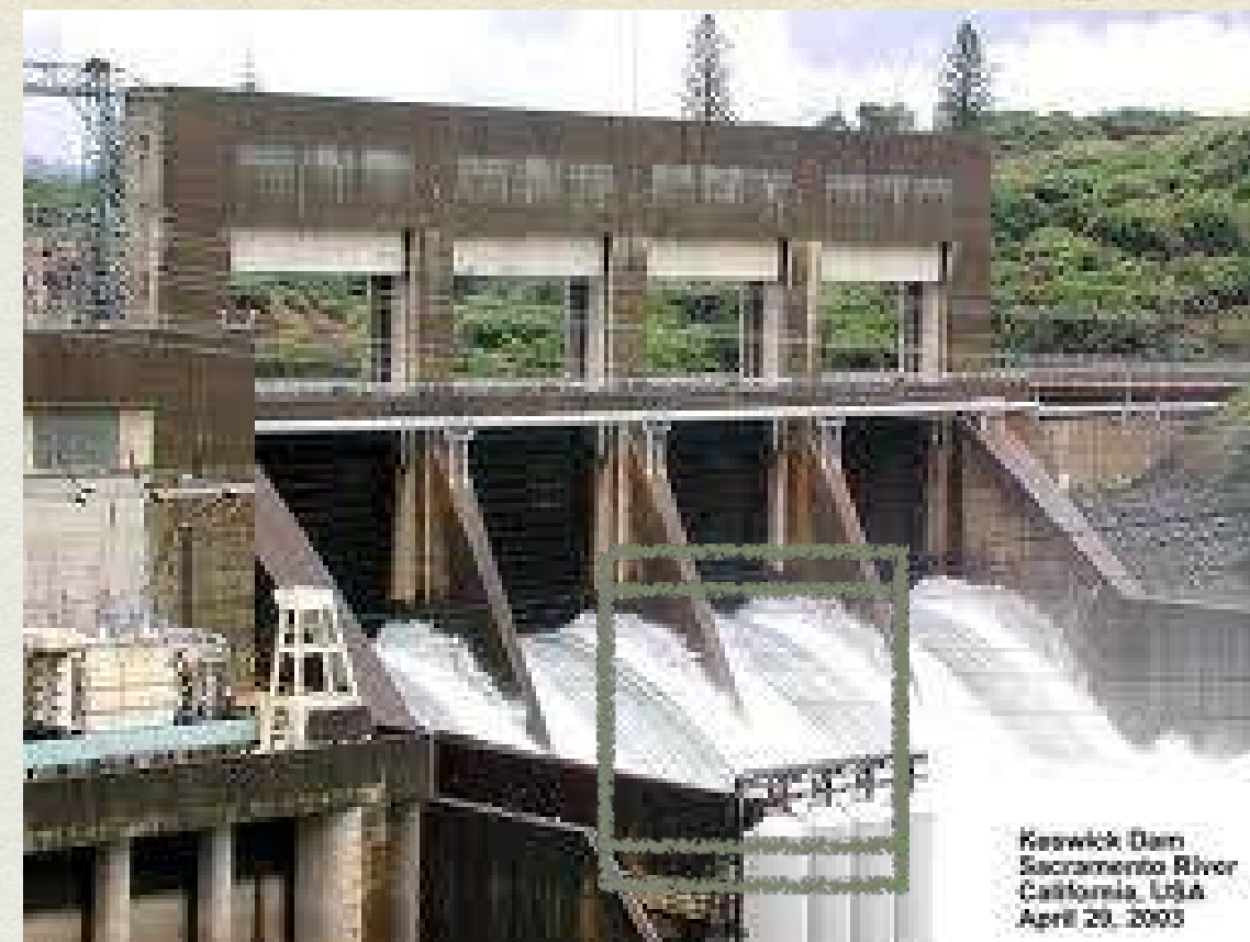
Keswick Dam - 3 miles north of Redding - completed in 1950
